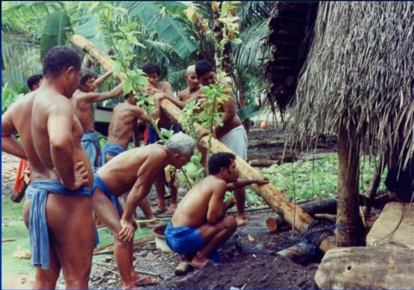
Canoe House Repair
